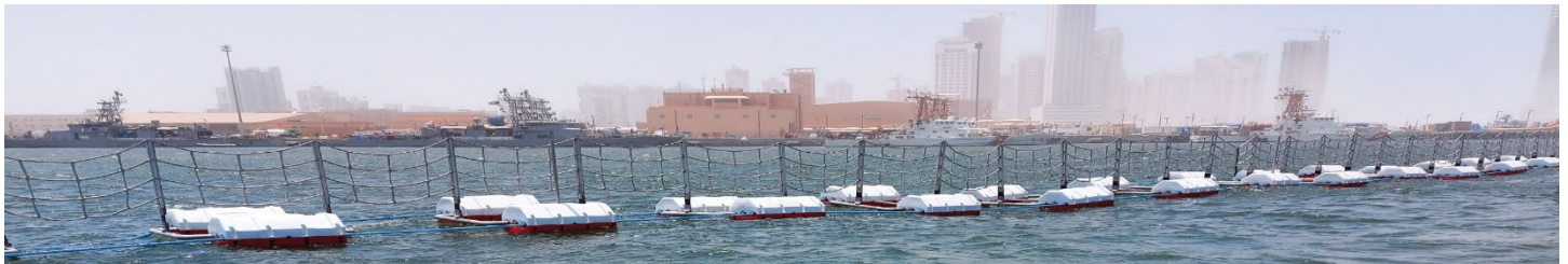
Port Security Barrier
